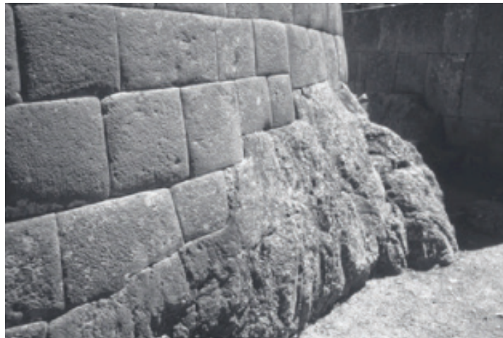
Figure 7: Building built on top of rock outcropping, Machu Picchu. Dean, Carolyn. Culture of Stone : Inka Perspectives on Rock. Durham [N.C: Duke University Press, 2010]
